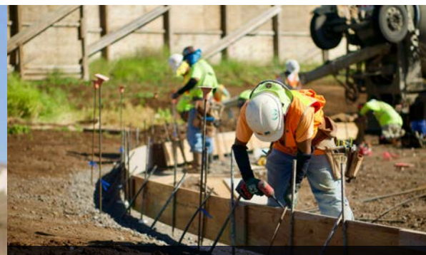
Apprentices work on state-projects to improve infrastructure.
