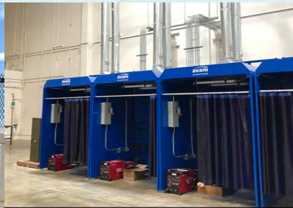
The Training Centers house top technology for training, including a several welding booths.
