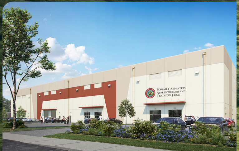
HCATF's new Training Center is the first facility on-island prepared to provide millwright training locally.
